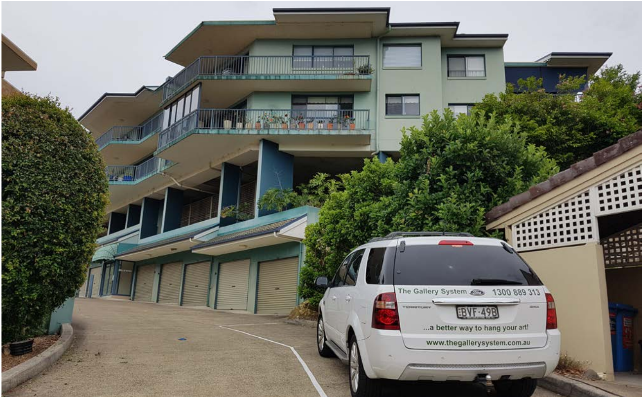
Figure 4 – View of existing seniors living units, Aveo Minkara
