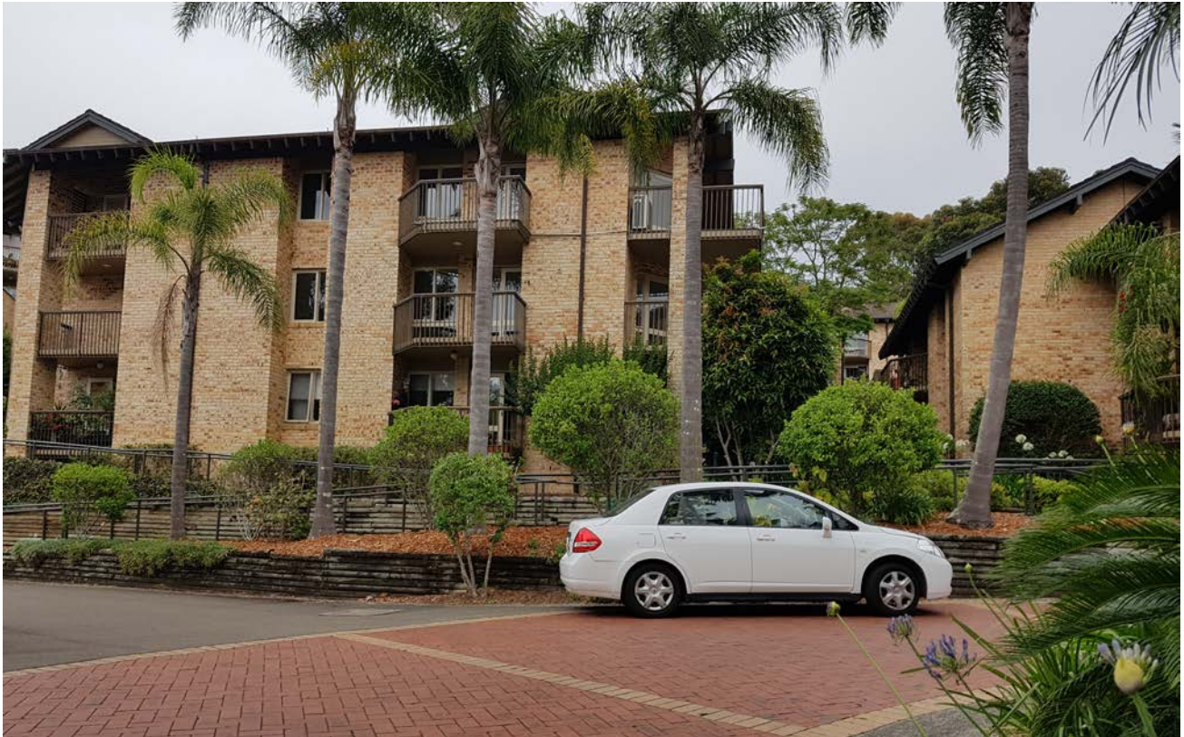
Figure 6 – View of existing seniors living units, Aveo Minkara
