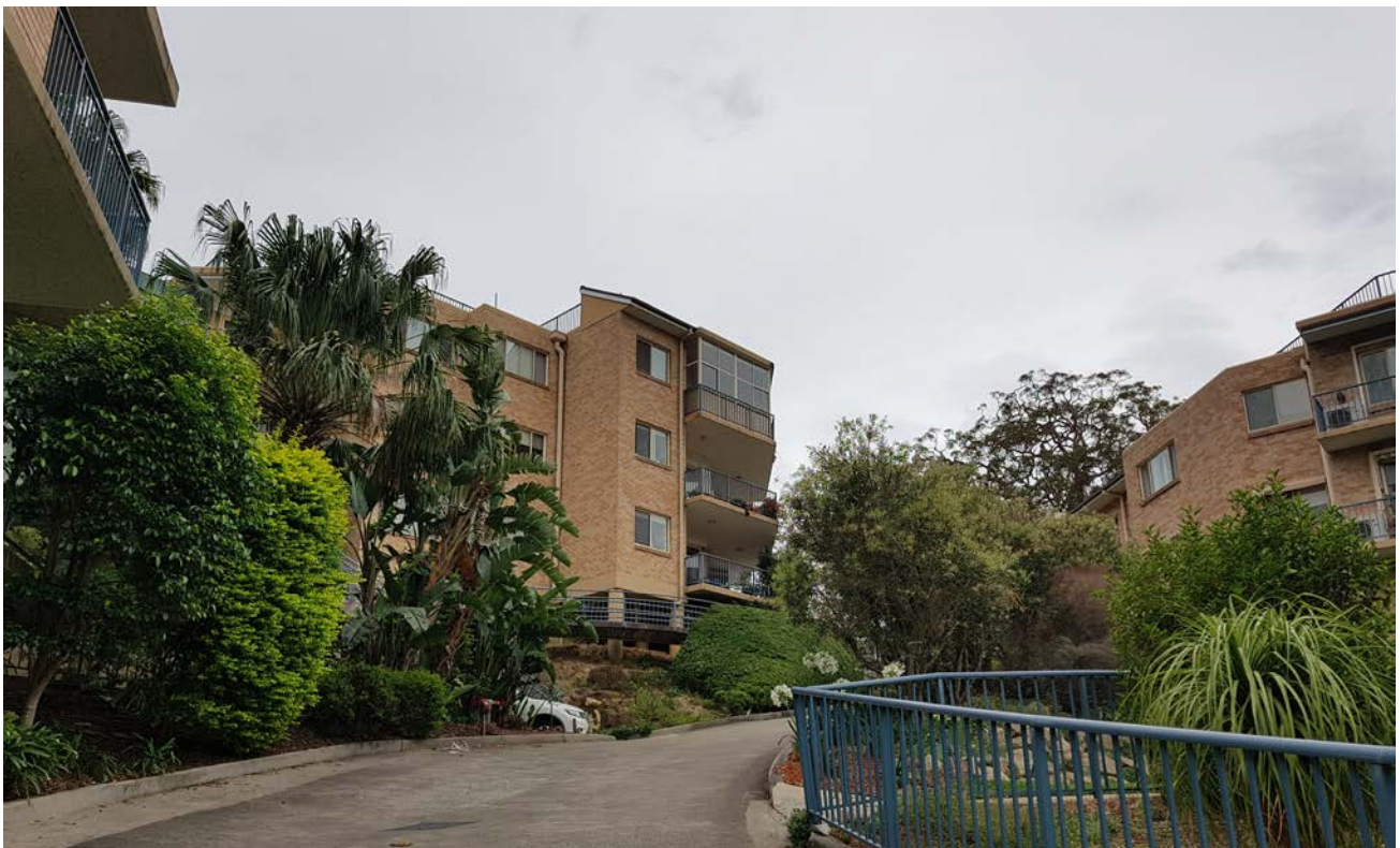
Figure 5 – View of existing seniors living units, Aveo Minkara
