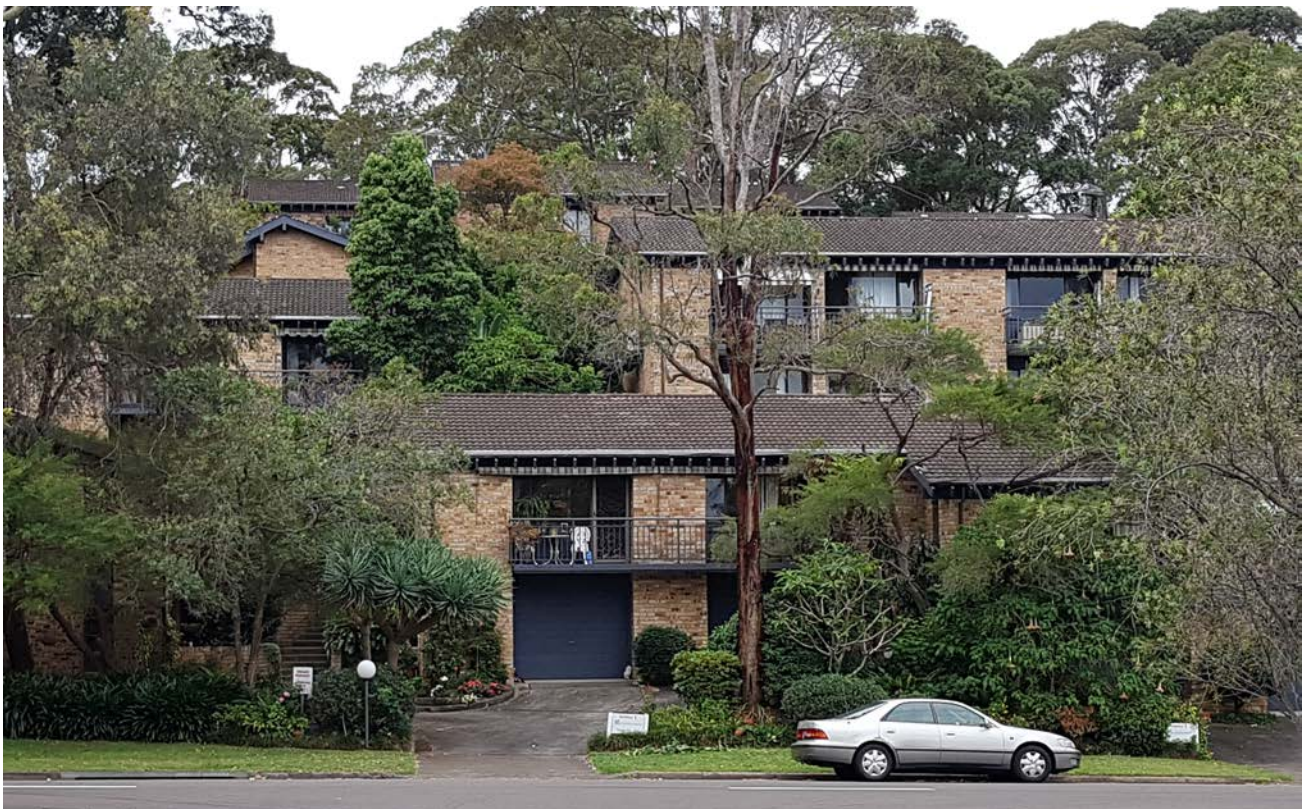
Figure 9 – View of existing seniors living units at Aveo Bayview Gardens, viewed from Kiah Close
